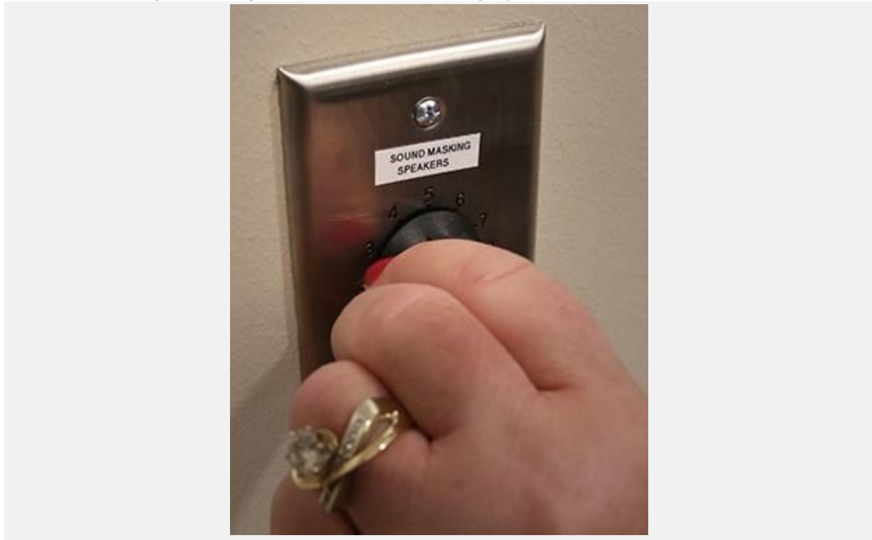
The most high-tech feature in Bremer Financial Corp.'s space is the SmartSMS-NET Sound Masking System, which produces "white" and "pink" noise. Staff photo: Bill Klotz
