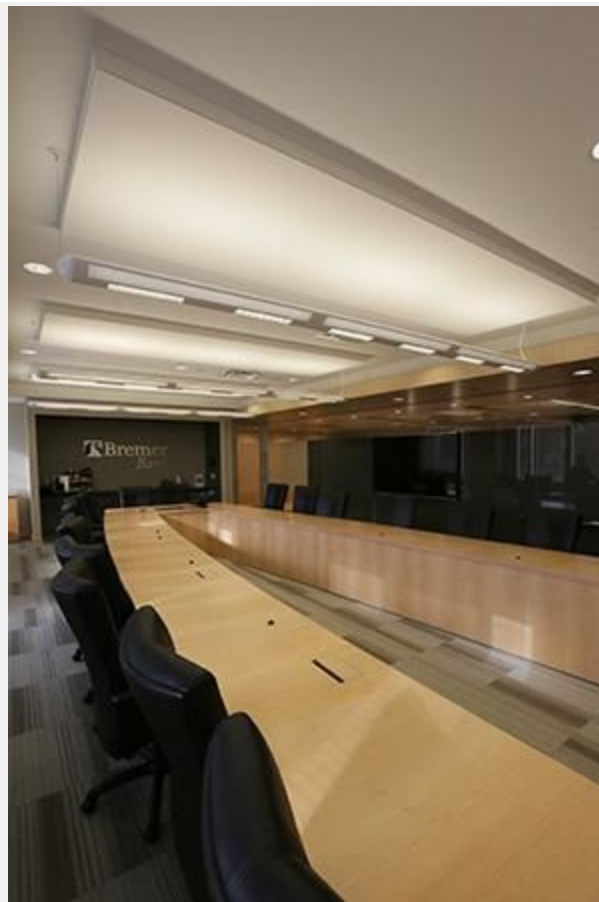
A SNAP-tex fabric wall and ceiling system designed to absorb sound extends along the walls and into the Bremer Financial Corp. boardroom. Staff photo: Bill Klotz
